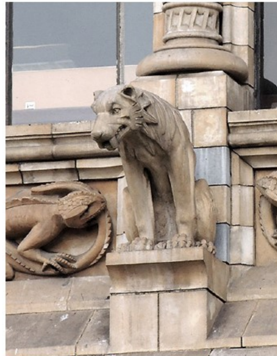
Ornaments in place; first floor windows, east-wing
